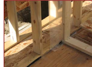
Double-stud 2x4 walls with Usi-0.10 (R-56) cellulibre
