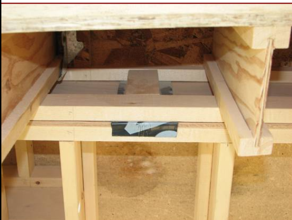
Spreader plate joints sealed
