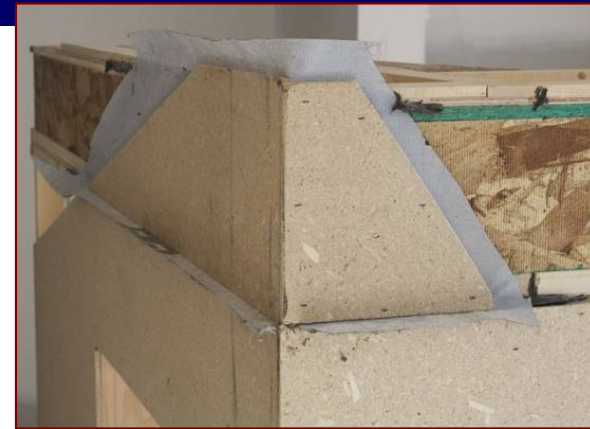
Rim joist air barrier wrap
