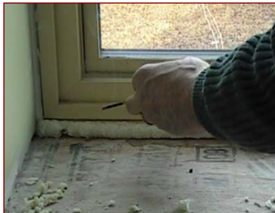
Windows foamed All penetrations sealed
