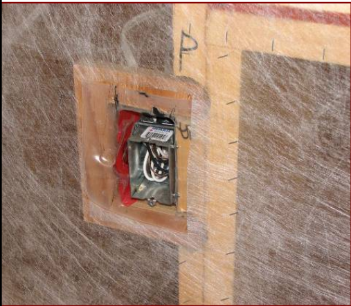
Electrical poly-vapour hats and backers
