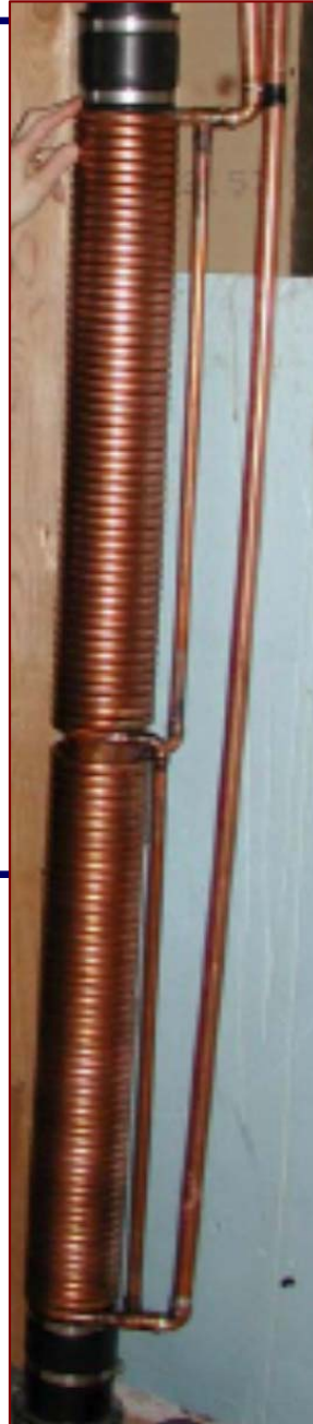
Drain water heat recovery
