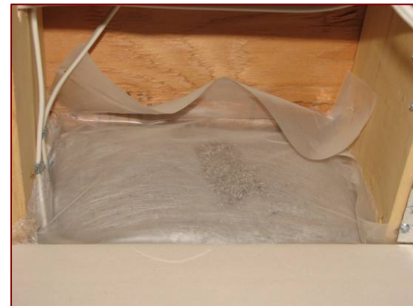
Rim joist vapour barrier
