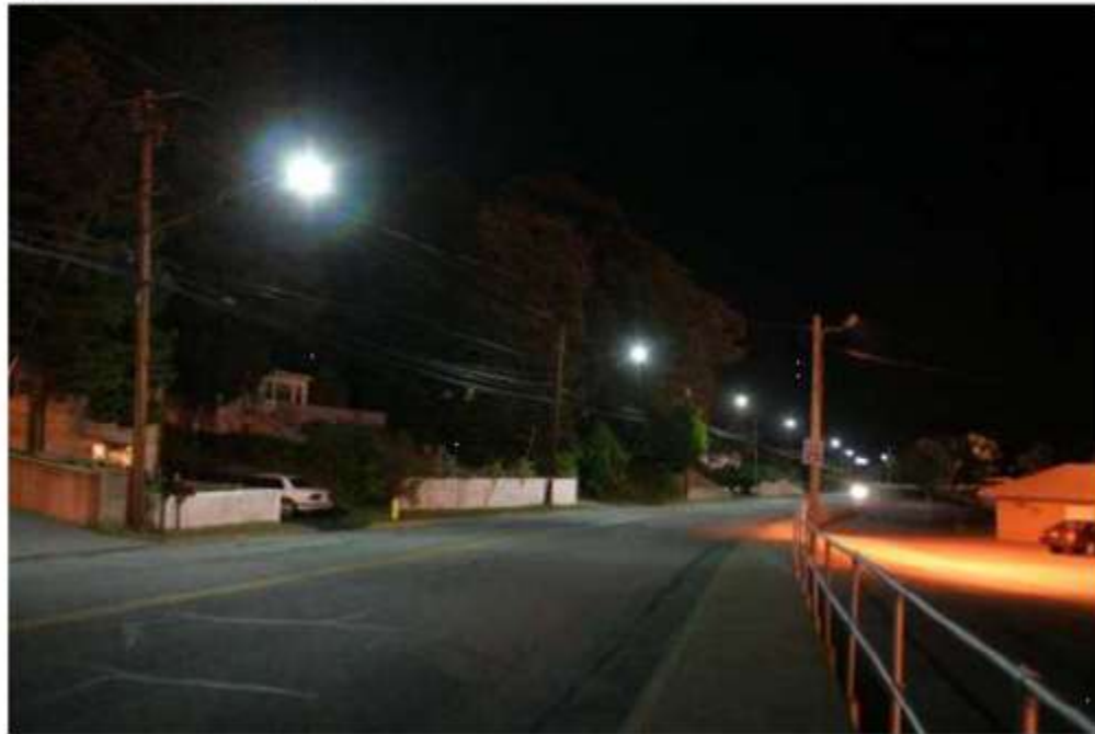
Figure 3. Induction street lighting demonstration (Meridian Street)
