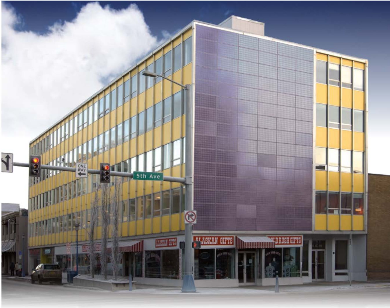
East Fifth Ave. – Vertical mount used as siding – The Solar Building – 17.28 kW
