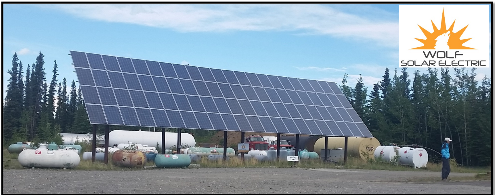
Grid tie off the Alaska HWY 4 in the town of Tok 23kw array at Northern Energy
