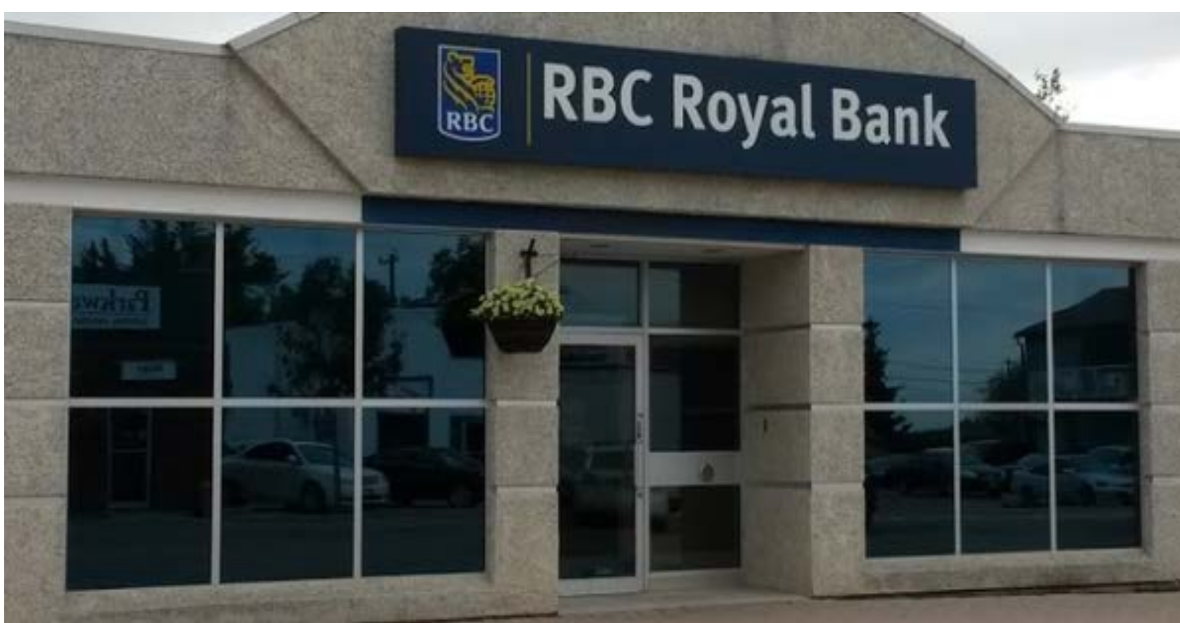
RBC Erickson, Mold remediation requiring major renovations
