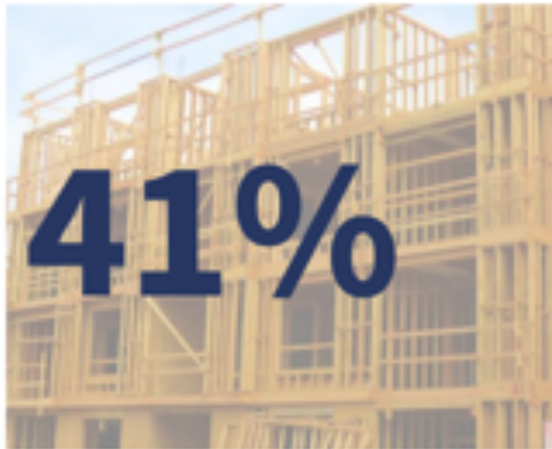
Wood-framing with concrete slab
