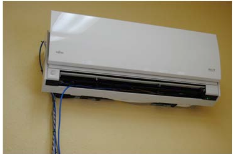
Ductless ASHP Interior Head
