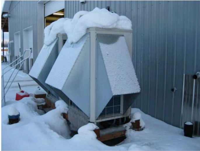
Outdoor coils of an ASHP in North Pole, AK
