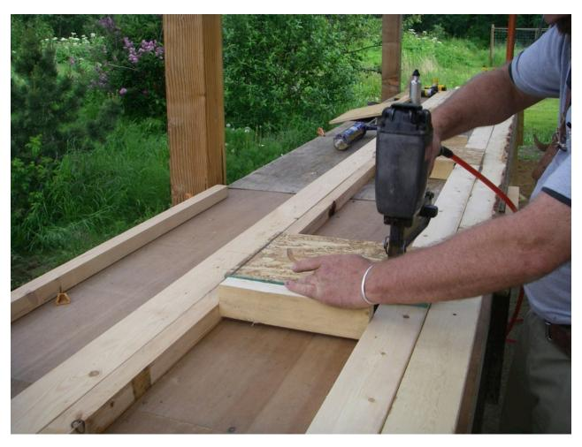
Gussets at 4-foot spacing – glued and nailed
