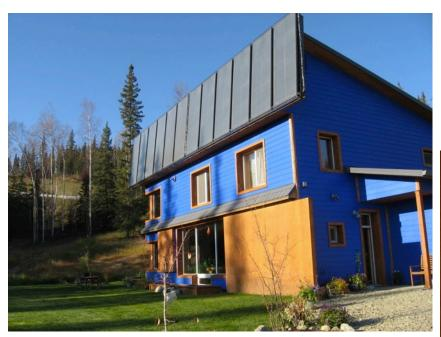
Solar thermal Flat-plate Collectors 5000-gallon thermal storage
