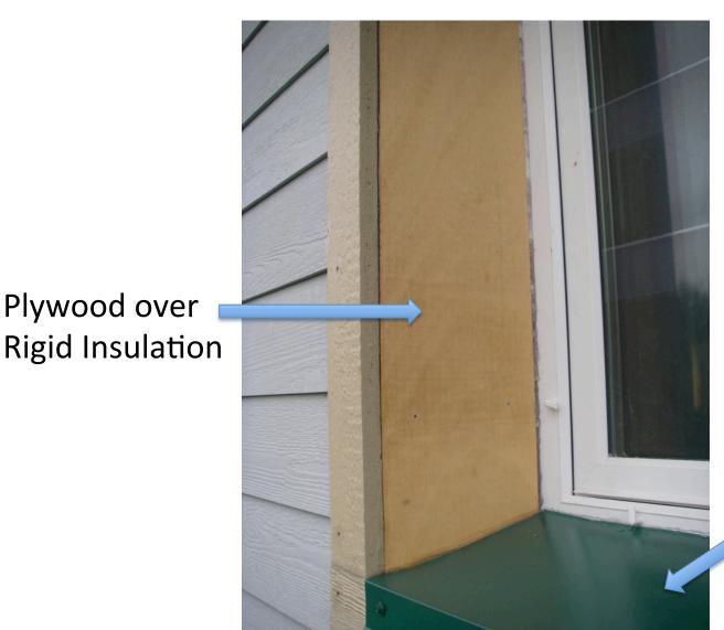
Sloped metal sill Over Rigid Insulation
