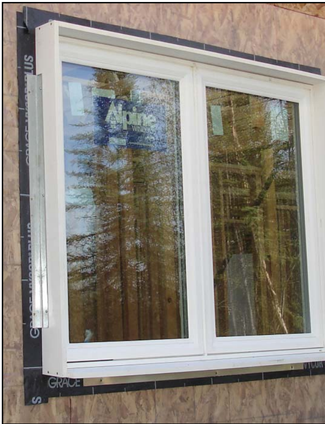
Image 13. Inset window with AZEK® jamb extension, attached to the sheathing using 2 inch x 2 inch light gauge galvanized flashing
