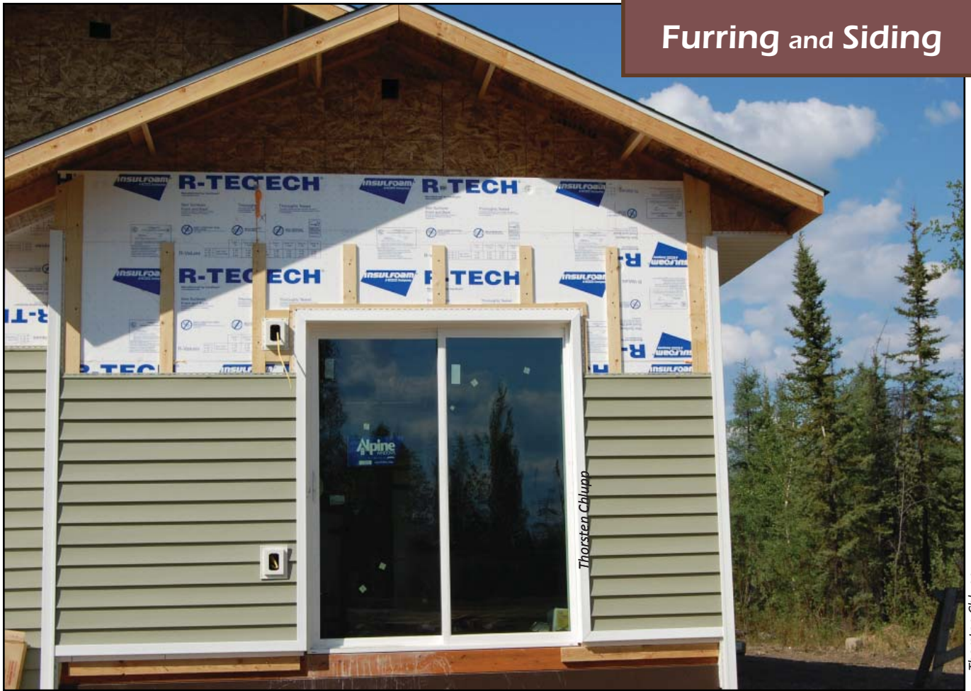
Image 36. Vinyl siding in progress
