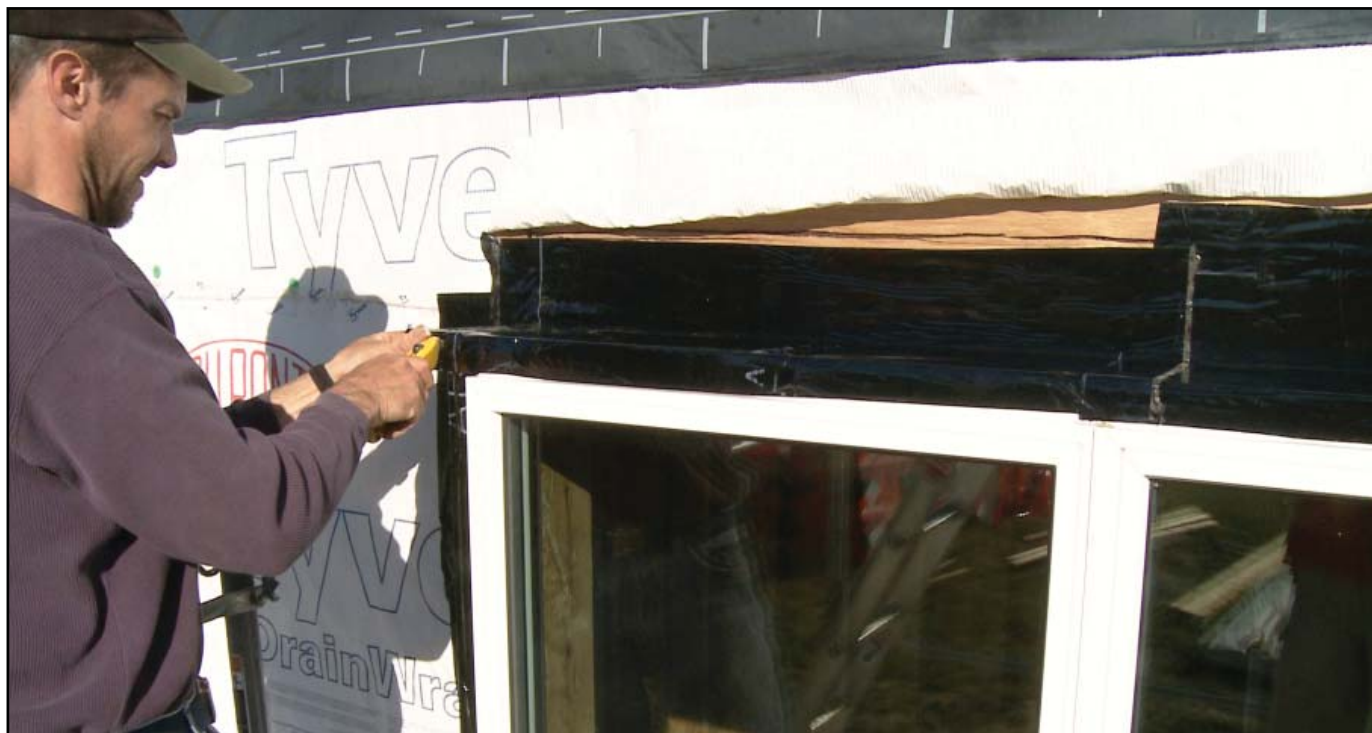
Image 11. Shingle-style flashing on exterior window buck
