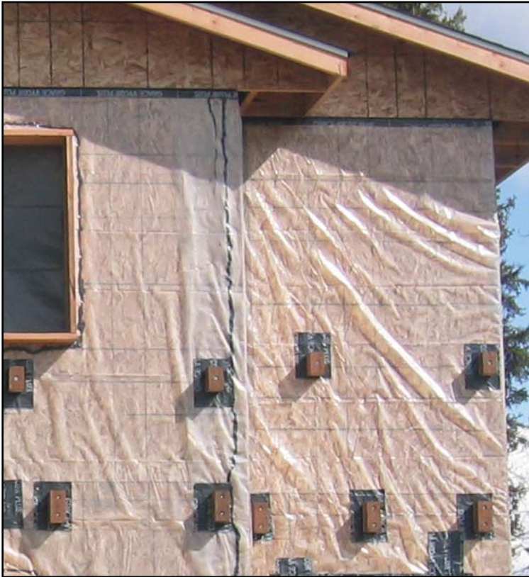
Image 3. Deck blocking over 6-mil polyethylene
