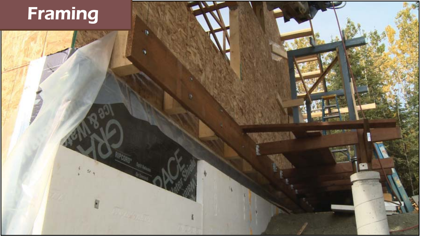
Image 6. Deck blocking and ledger board
