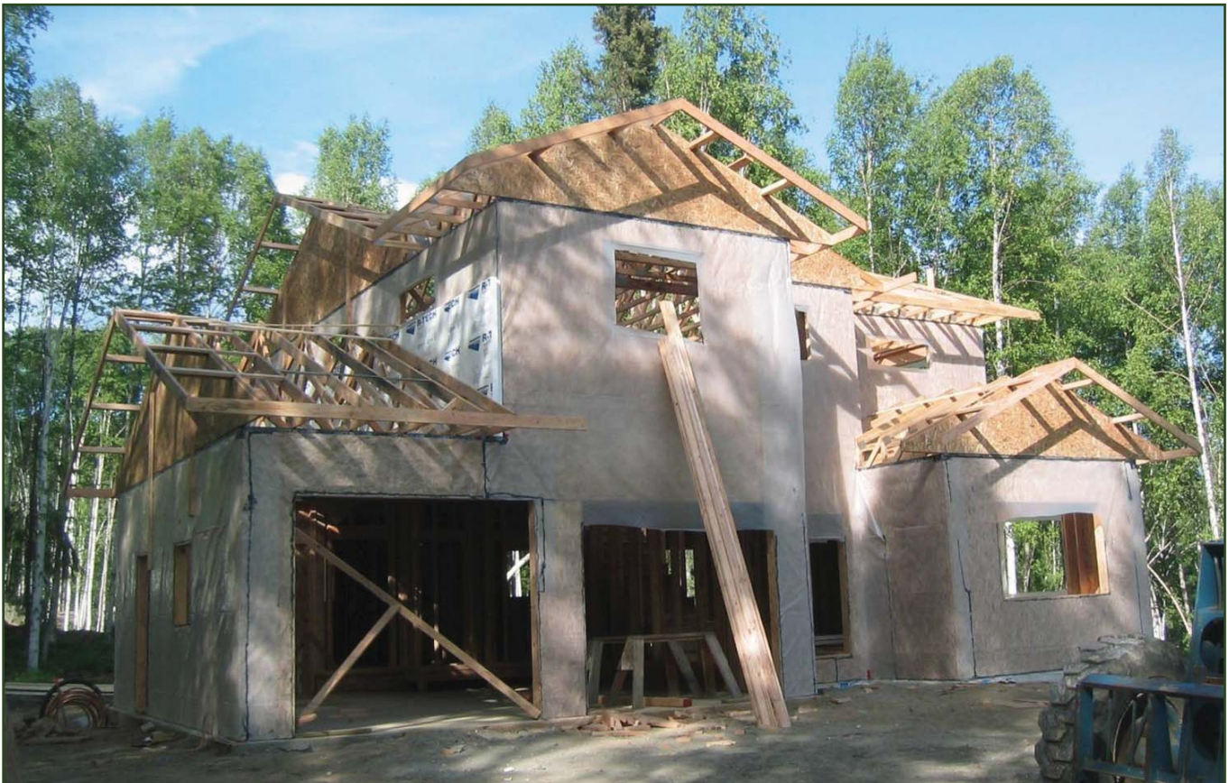
Image 20. 6-mil polyethylene exterior vapor retarder, note installation of foam board against wall before installation of garage gable truss
