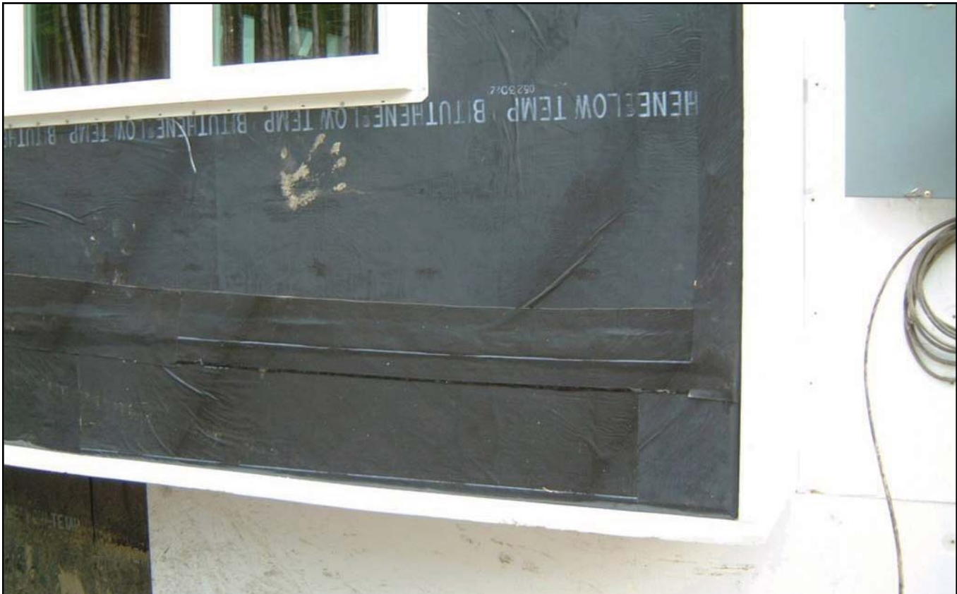
Image 28. Close-up of a square cantilever bay window with attached foam board
