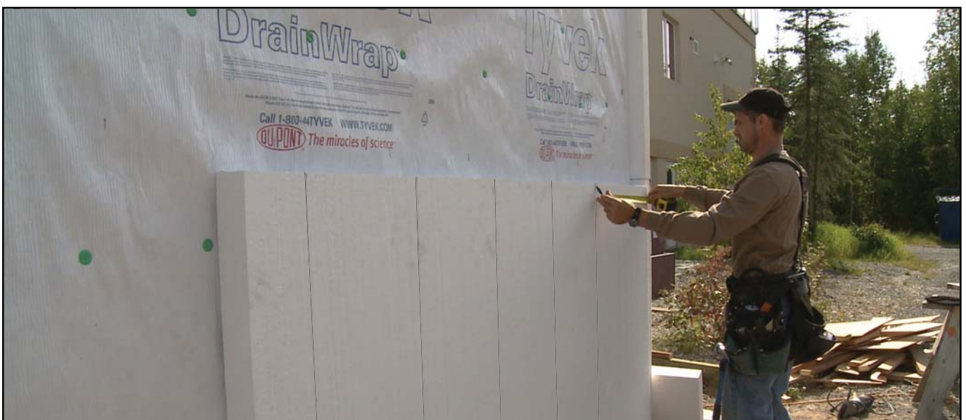
Image 25. Attaching first layer of foam board and transferring underlying stud pattern to the exterior foam board
