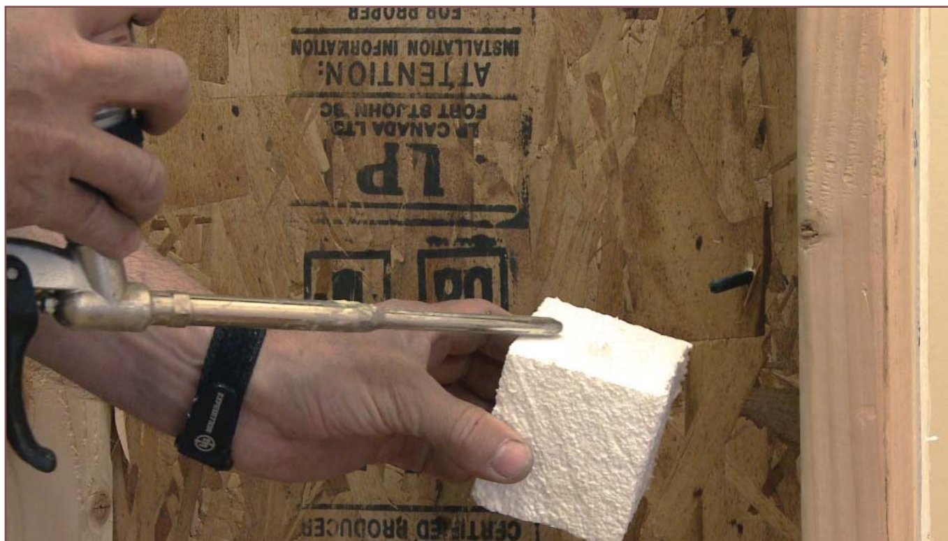
Image 32. Exposed fasteners inside the wall must be covered to prevent condensation
