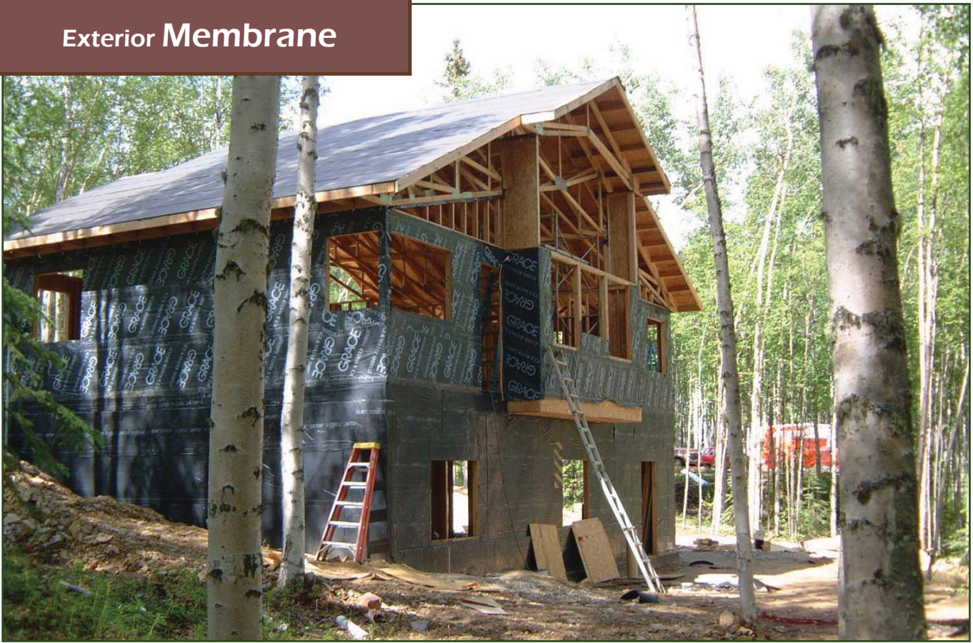
Image 19. Grace Bituthene® exterior membrane, one of several vapor retarder options
