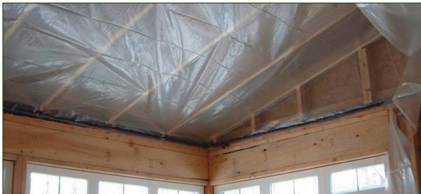
Image 24. Transition of interior ceiling vapor retarder to membrane strip on double top plates
