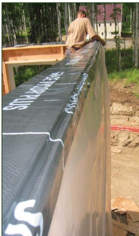
Image 22. Adhesive strip detail
