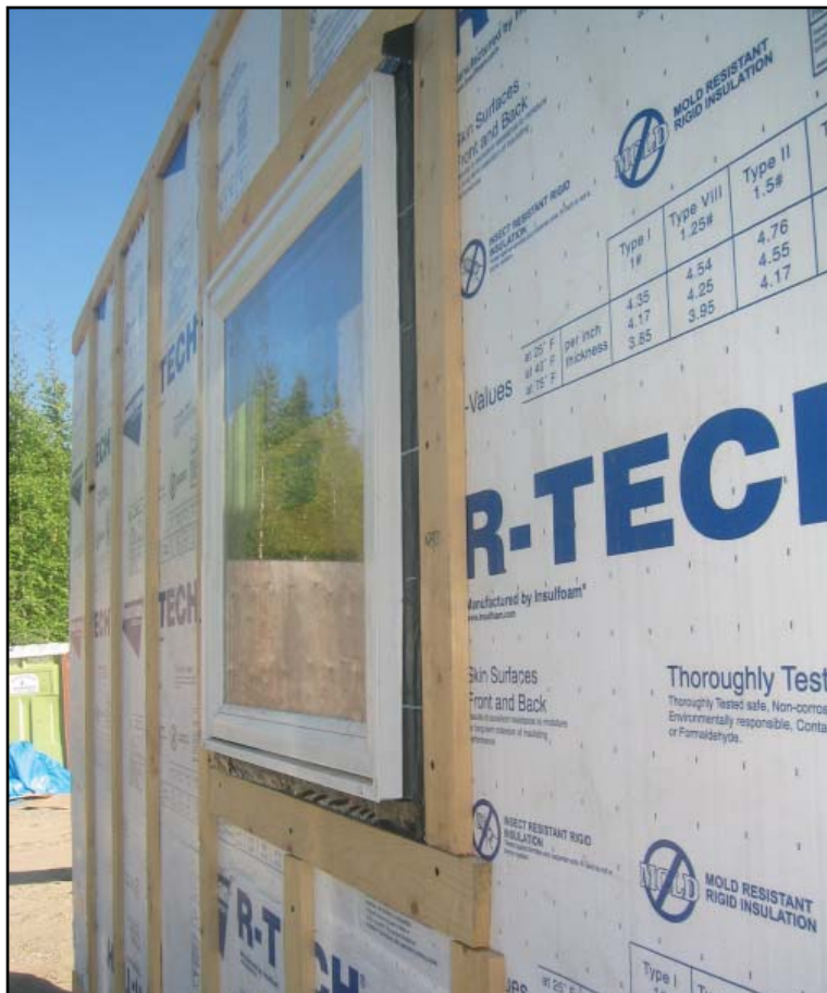
Image 34. Furring wraps around the window buck edges so that the window can seal directly to the membrane on the buck
