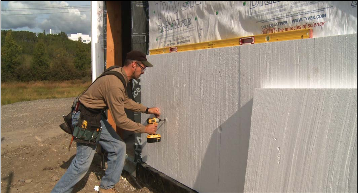
Image 26. Foam board is loosely attached to framing with a four inch sheetrock screw and a Wind-Lock® plastic washer
