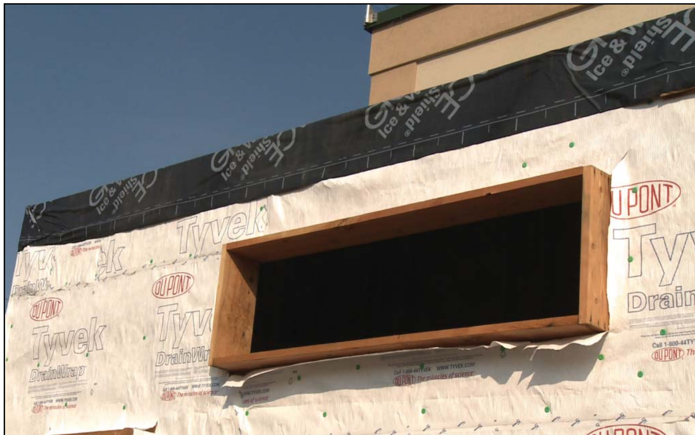
Image 8. Tyvek® DrainWrap™ is showing promise as an exterior membrane option, (as pictured here and the following pages on the CCHRC facility). It has met with code approval in areas of southeast Alaska, and its performance during sustained periods of extreme cold continues to be tested in Fairbanks.
