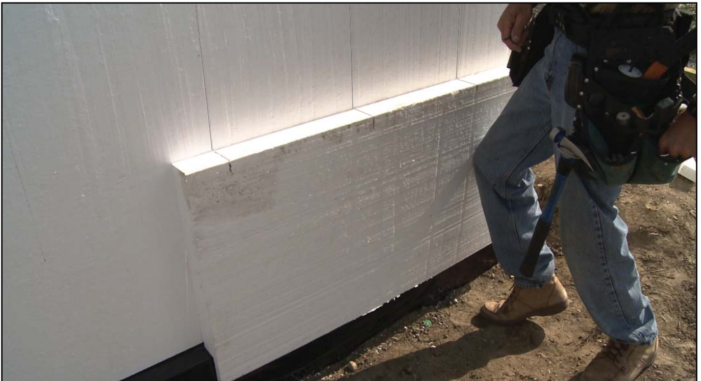
Image 27. Second layer of foam board is loosely attached using transferred stud pattern with eight inch screws and Wind-Lock® washers
