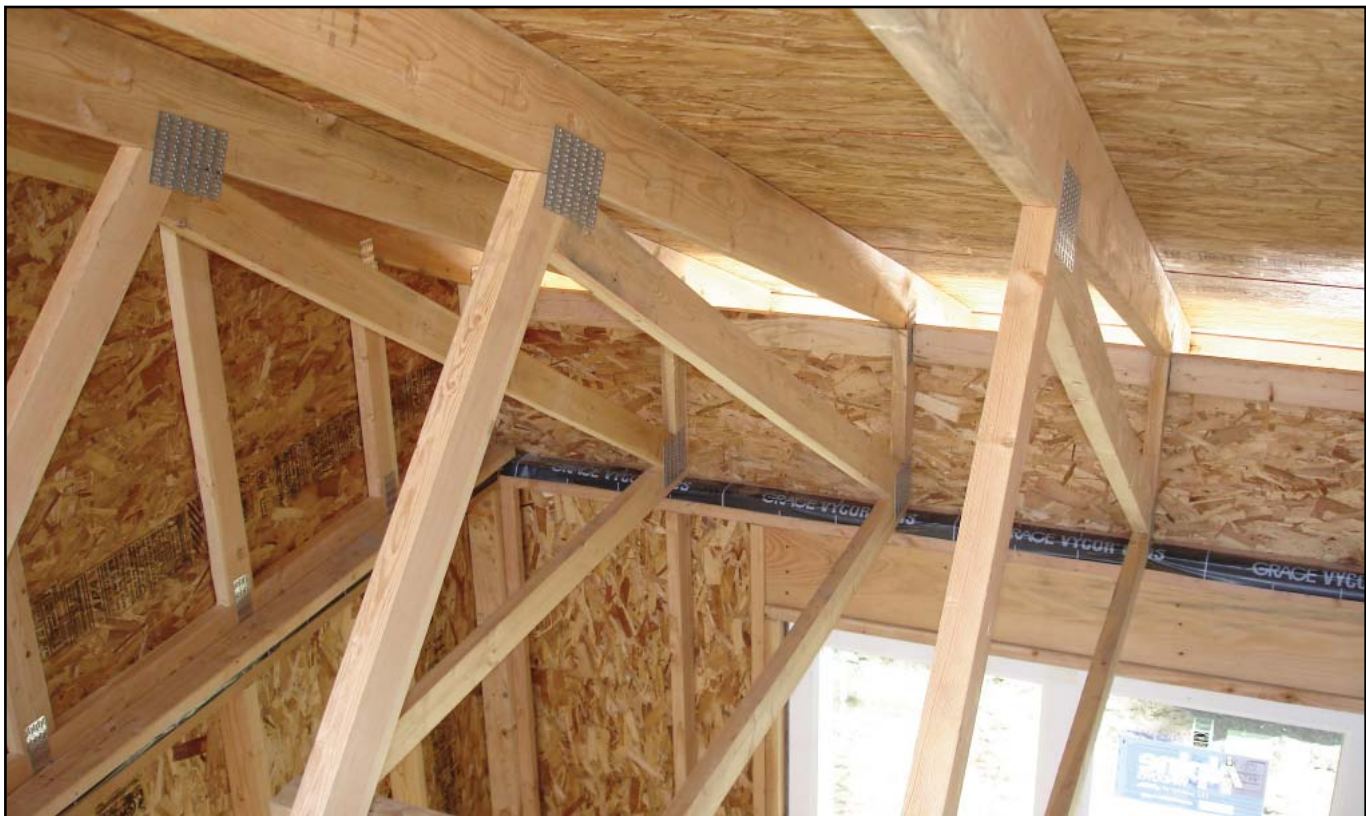
Image 2. Interior View: 18-inch-deep energy heel truss allows for R-60 roof insulation and easy continuation of wall foam to the top of the attic insulation
