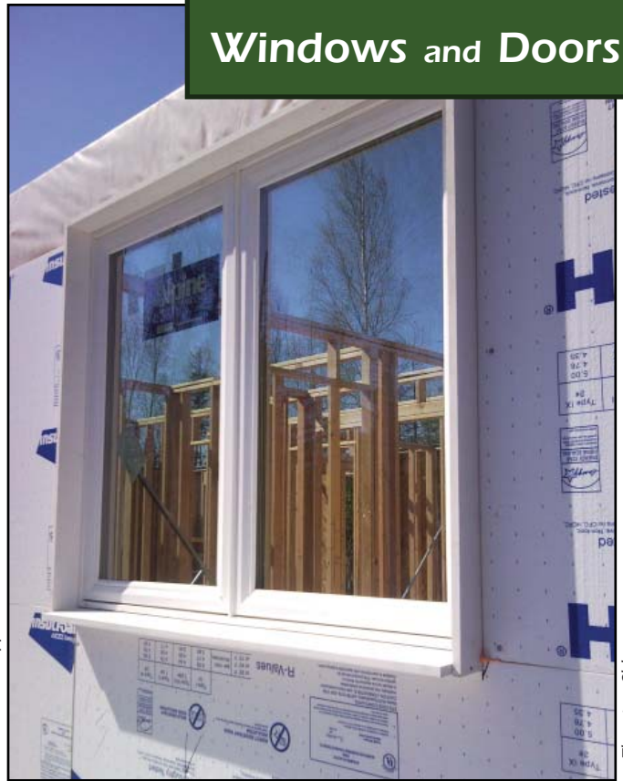
Image 14. Inset window with AZEK® and first layer of foam
