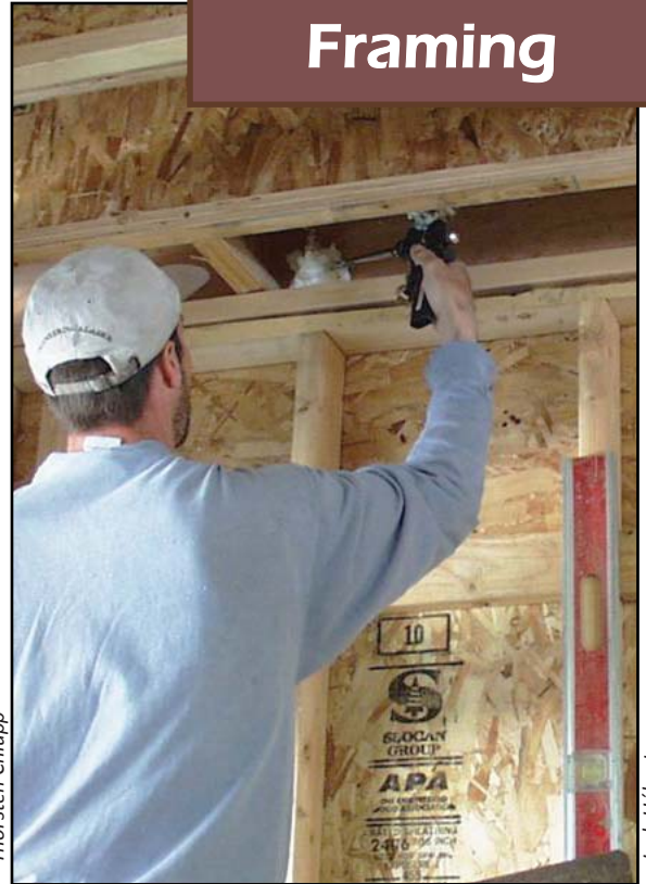
Image 4. Insulating deck fastener penetrations on interior to prevent condensation
