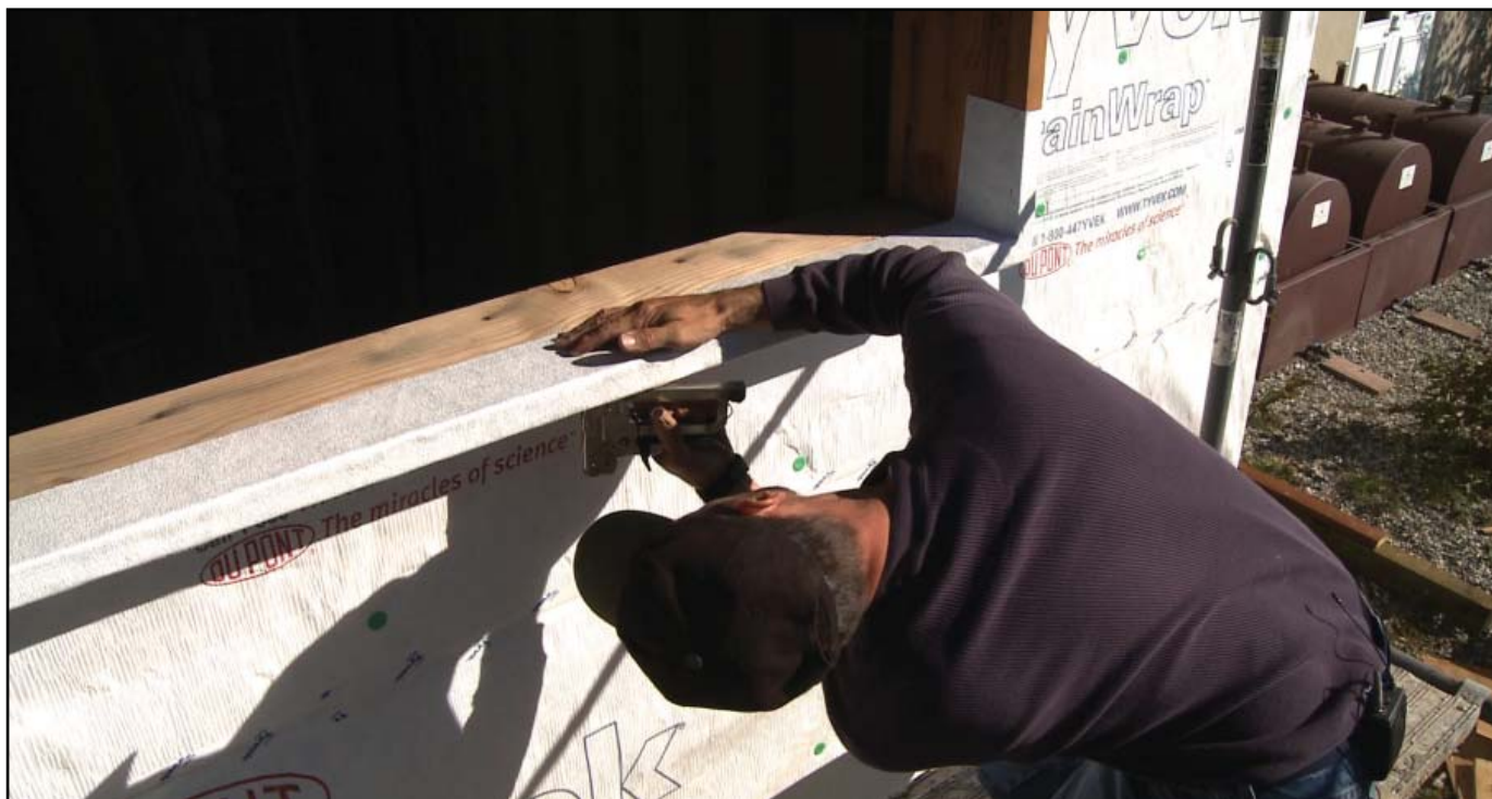
Image 10. Exterior window buck sill corner detail. Tyvek® FlexWrap™ (or similar product) must be stapled around edges
