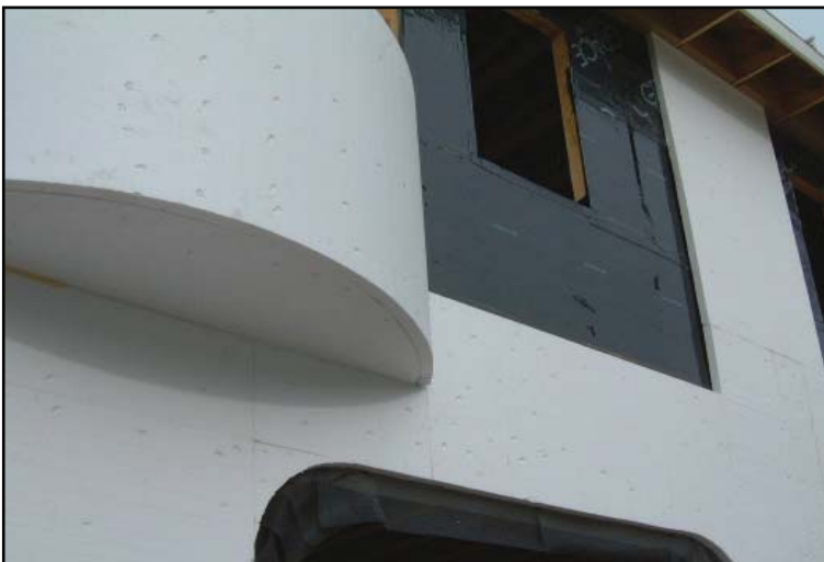
Image 29. Foam board covering a curved cantilever
