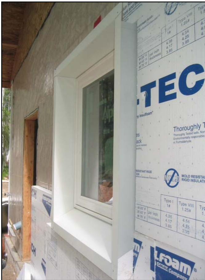
Image 15. Inset window with steel jamb extension
