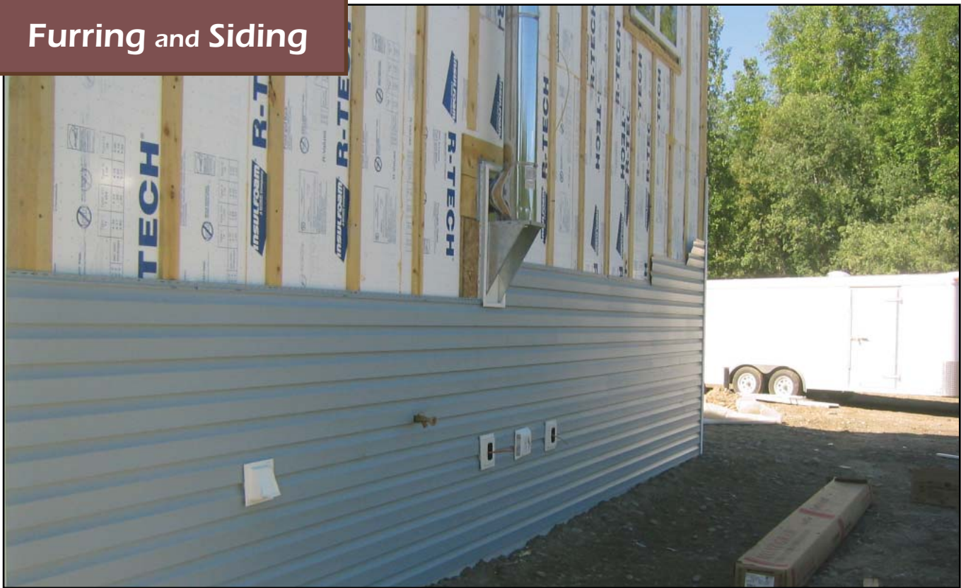
Image 33. Vinyl siding in progress, note furring around chimney support
