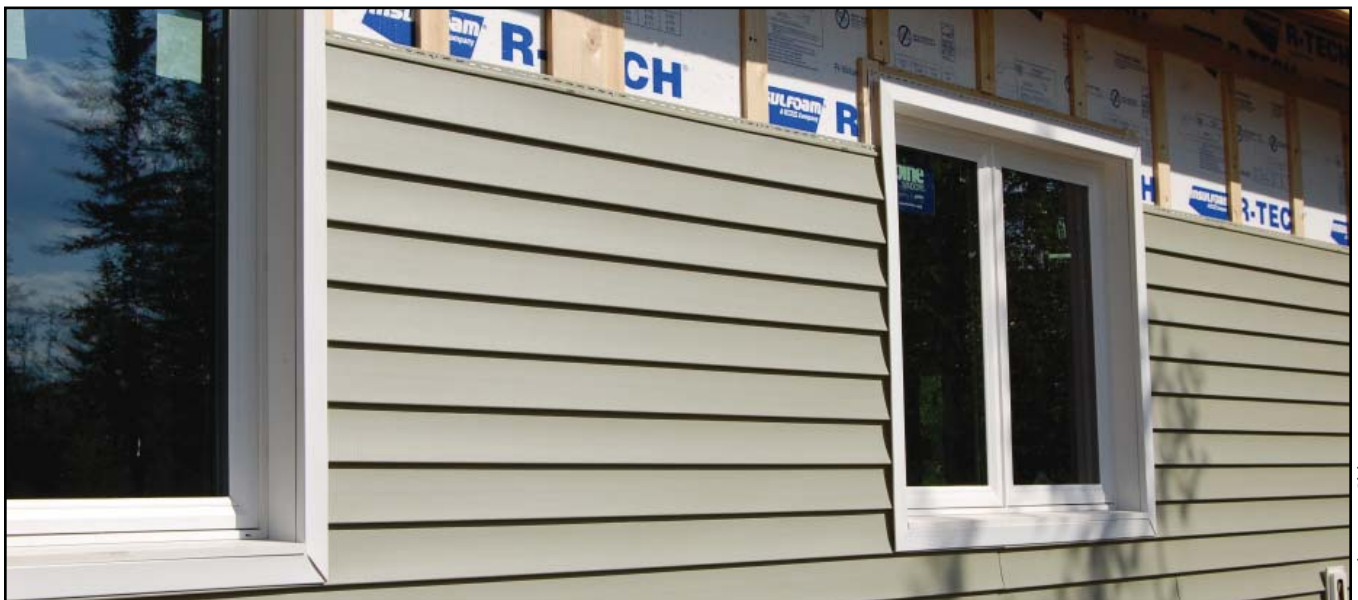
Image 12. Vinyl siding around inset window with AZEK® jamb extension
