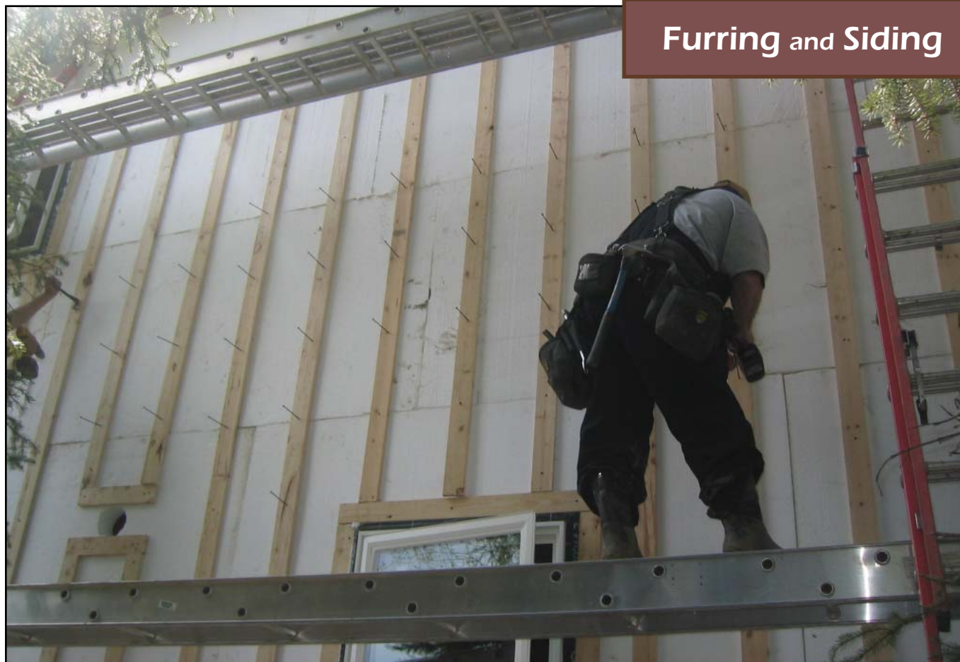
Image 31. Pre-drilled furring speeds installation process and keeps fasteners at a consistent height to avoid conflict with interior mechanical runs through the stud bays
