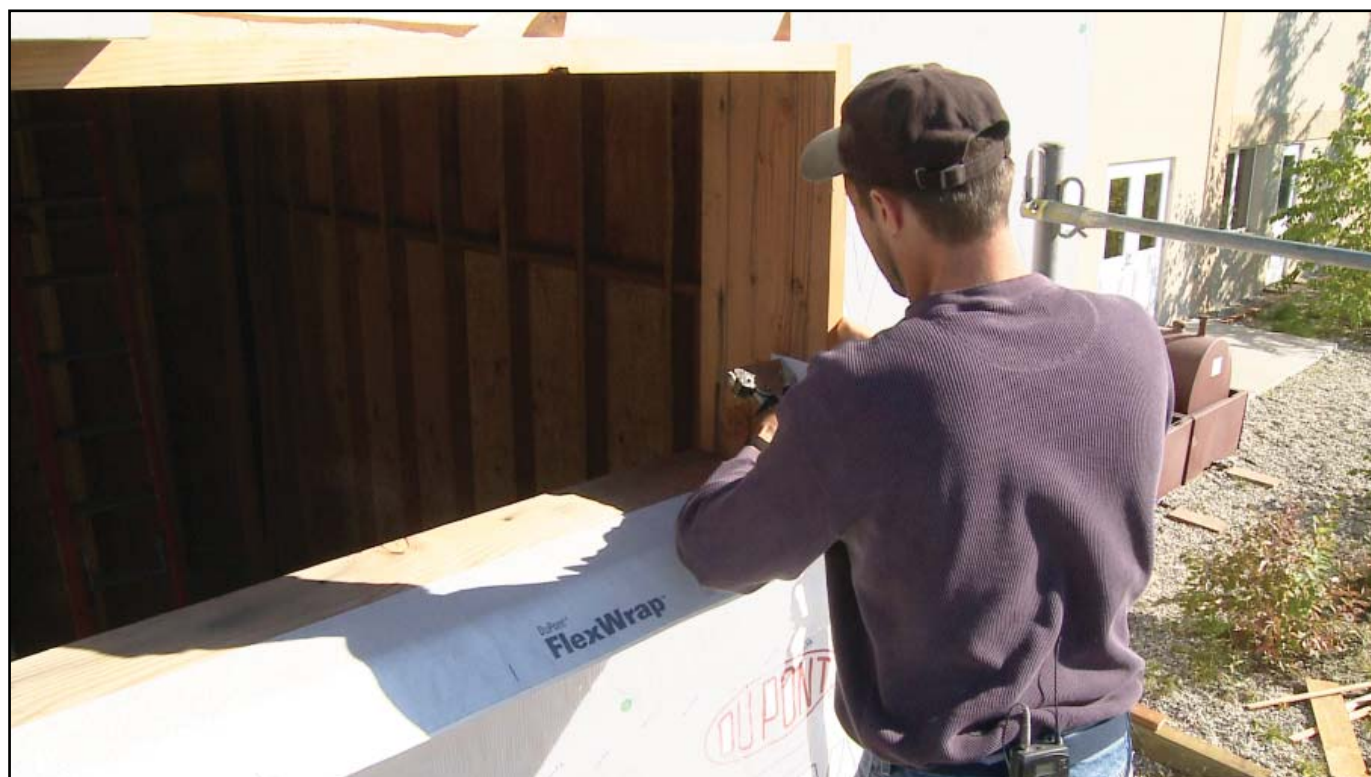
Image 9. Window buck sill detail with Tyvek® FlexWrap™
