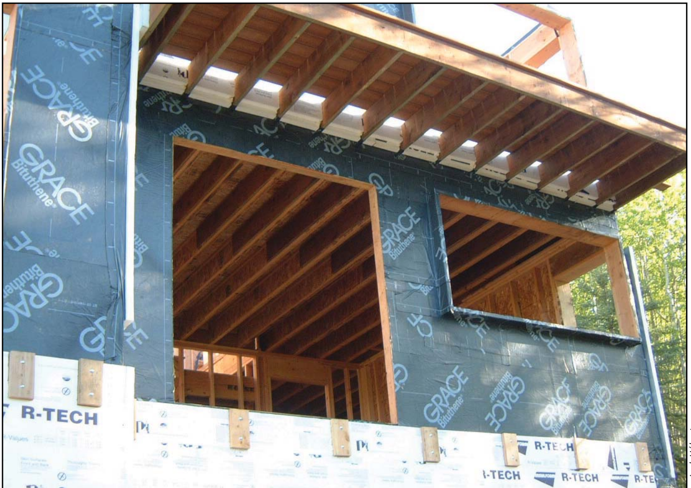
Image 5. Installed foam between cantilevered joists
