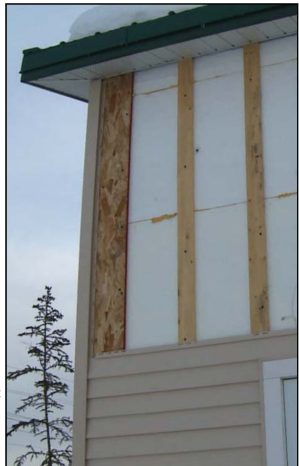
Image 35. Detail of wider furring on corner, allows for fastening to corner framing
