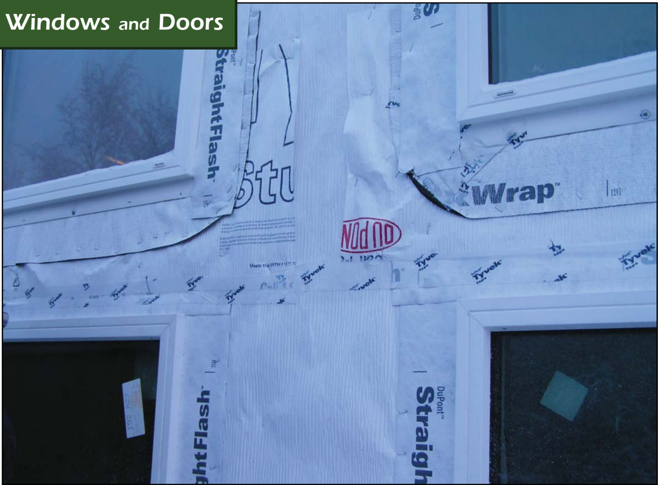
Image 17. Stucco preparation: Inset window flashing
