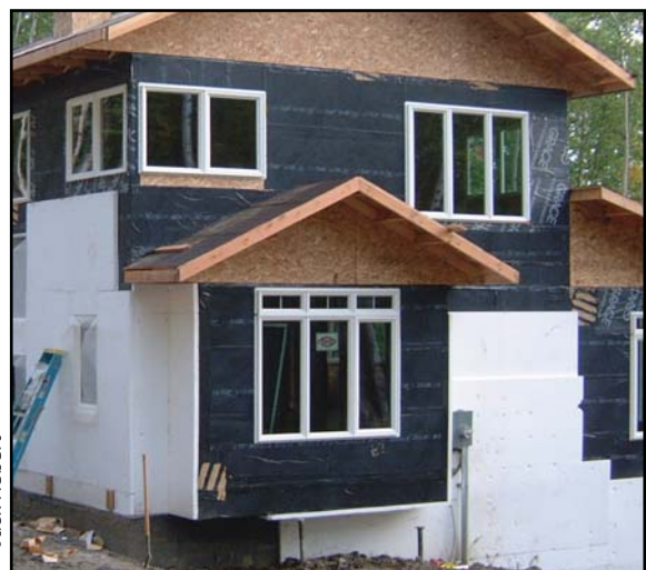
Image 30. Cantilevered addition wrapped with foam board
