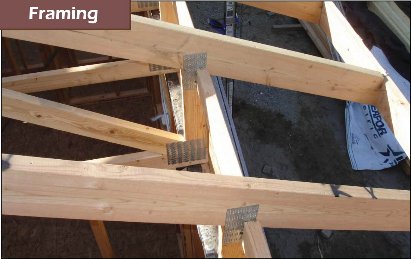
Image 1. Exterior View: 18-inch-deep energy heel truss allows for R-60 roof insulation and easy continuation of wall foam to the top of the attic insulation
