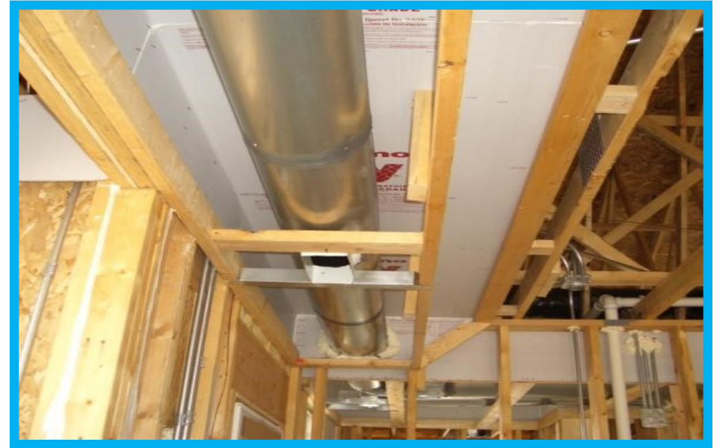
Seams and penetrations of air barrier properly sealed
