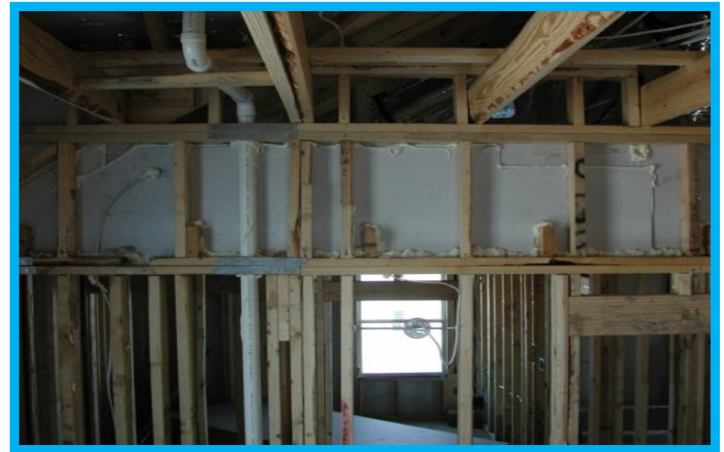
Backing air sealed prior to insulation.
