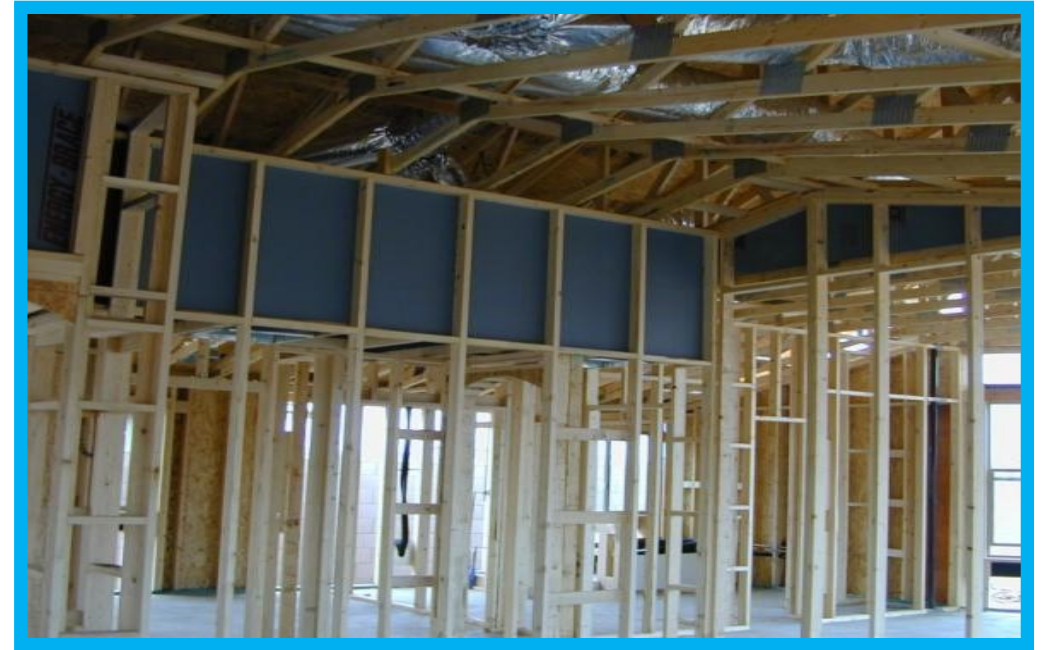
Rigid backing installed prior to insulation.
