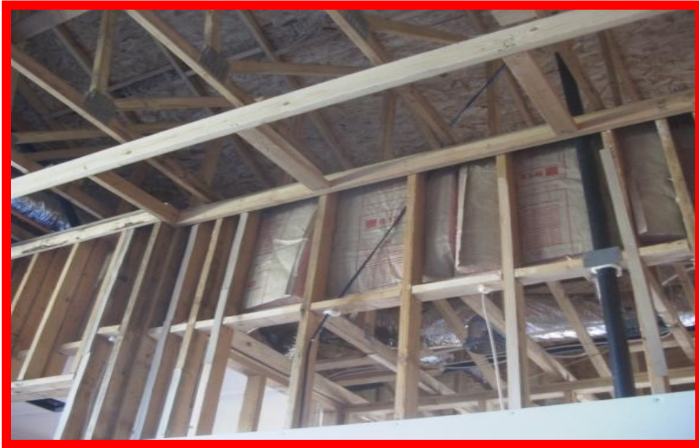
No rigid backing on knee wall.
