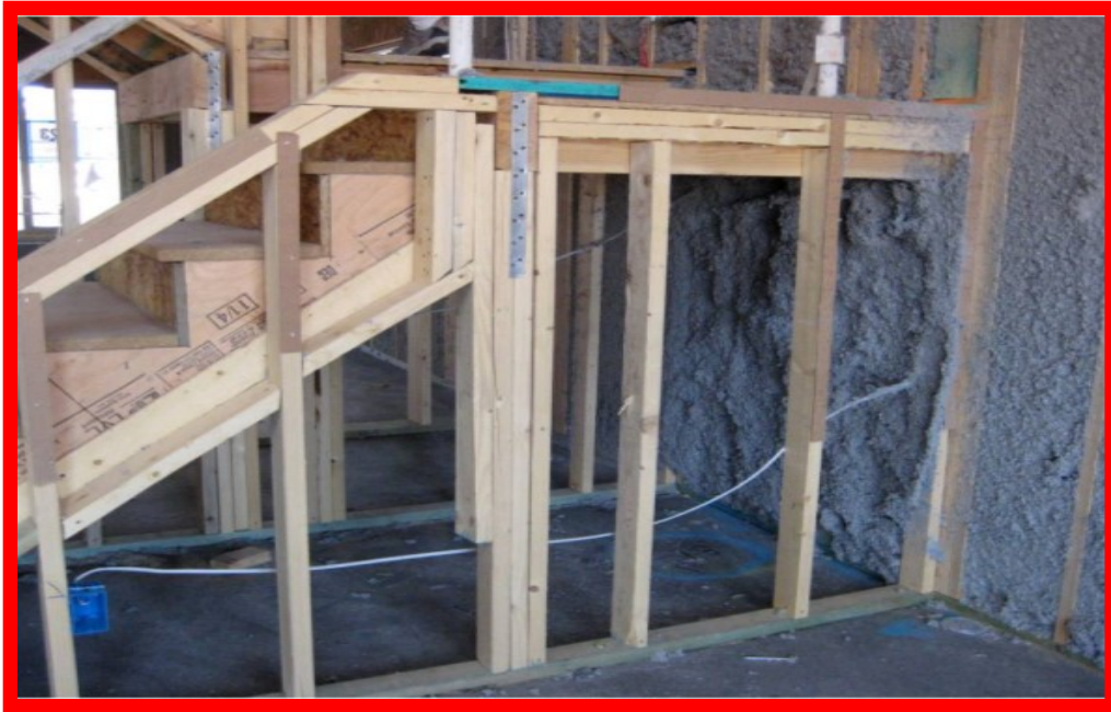
No air barrier installed under staircase.
