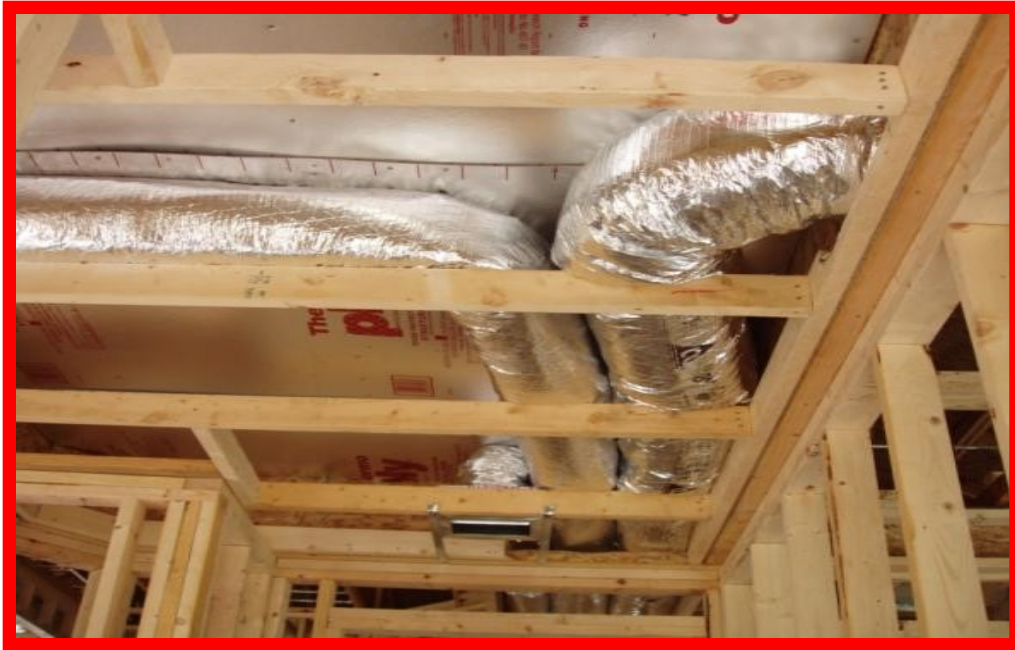
Seams of air barrier not sealed.
