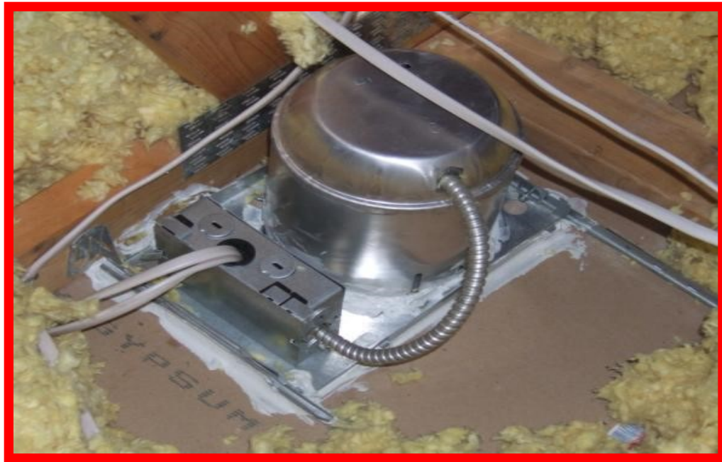
Non ICAT recessed light installed.
