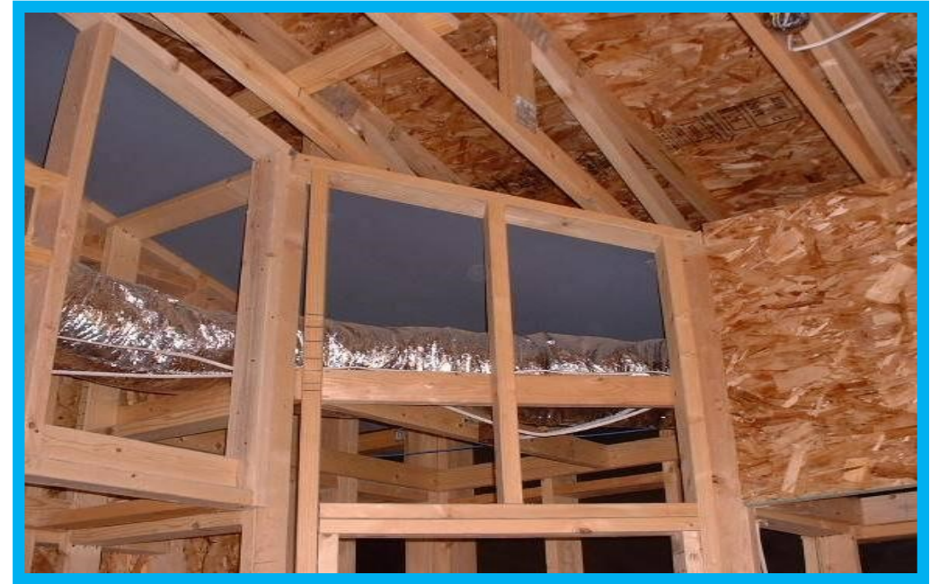
Air barrier is present between the dropped ceiling/soffit and the attic
