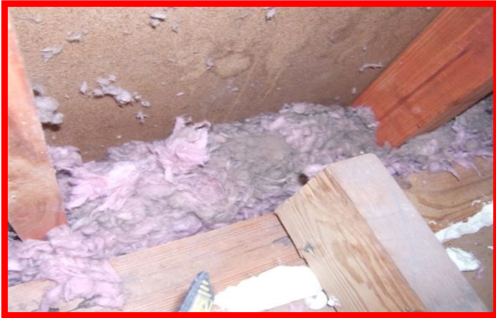
Wall from above without top plate or blocking installed.
