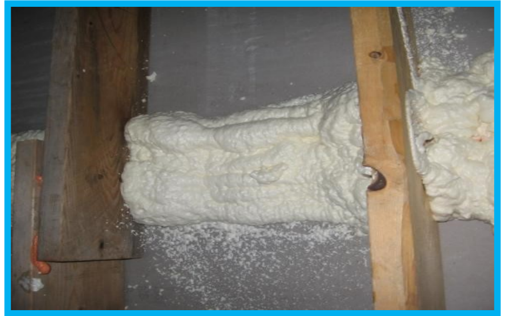
Top plate to drywall connection sealed from attic with foam.
