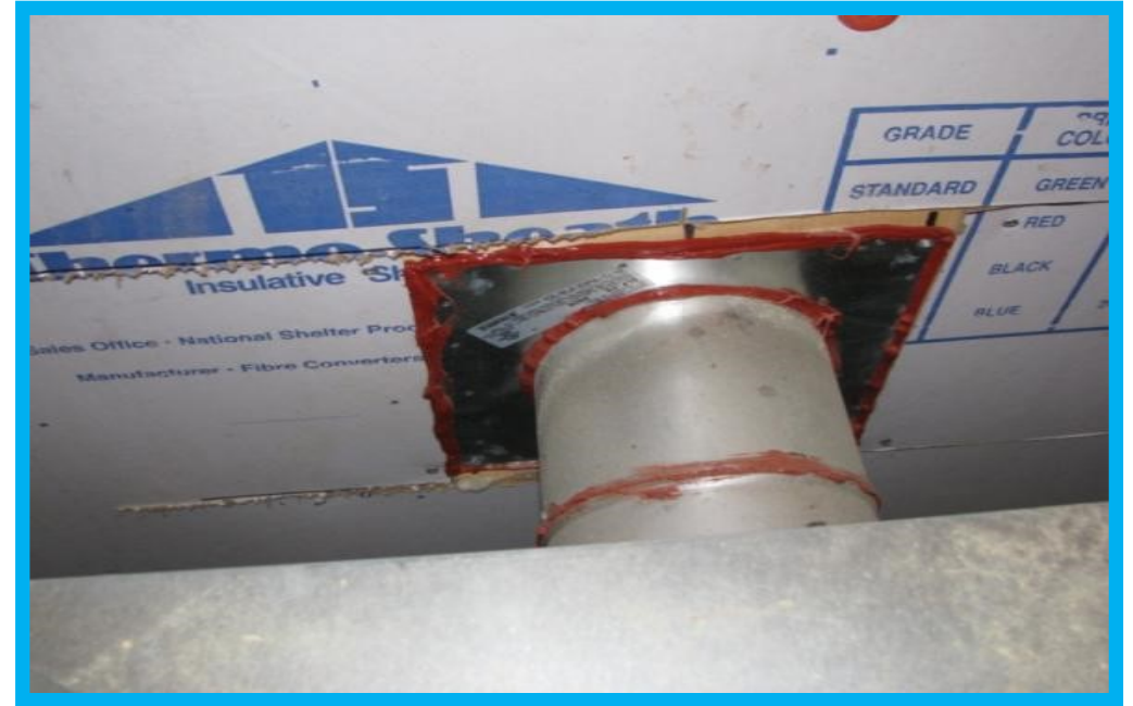
Vent and air barrier sealed.
