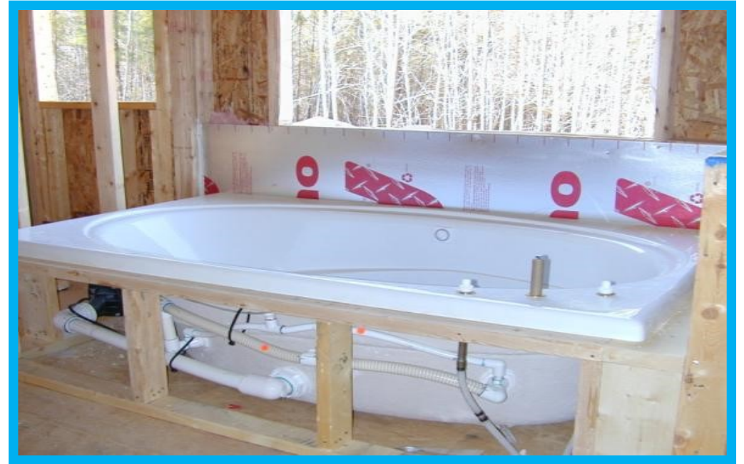
Air barrier installed behind the tub.
