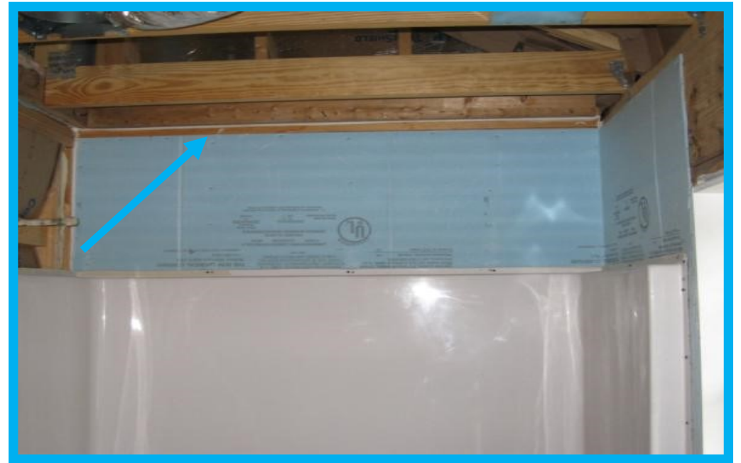
Air barrier sealed.
