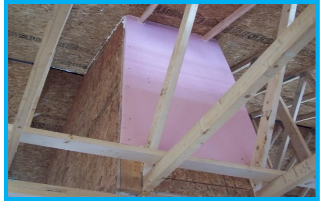
Rigid air barrier is installed to hold insulation in place.
