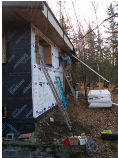
South wall insulation before new windows
