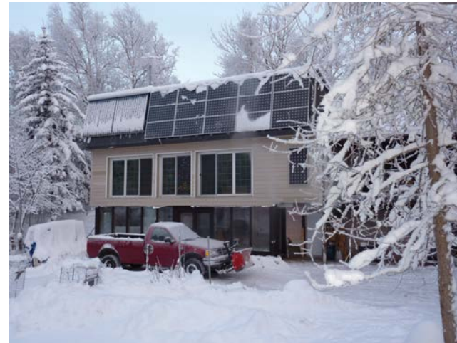
South view – December 2012 60,000 btu solar thermal 3 KW solar PV
