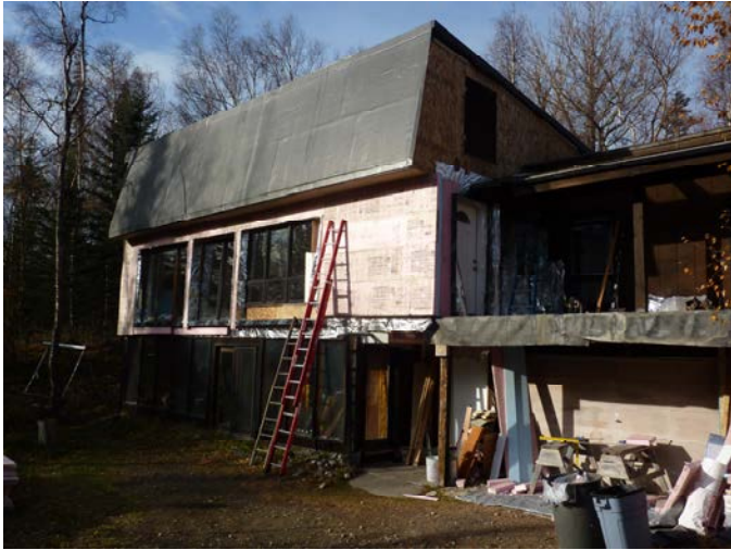
South wall insulation before new windows
