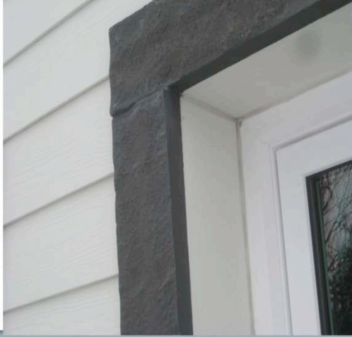
Cement Board for Inset window buck
