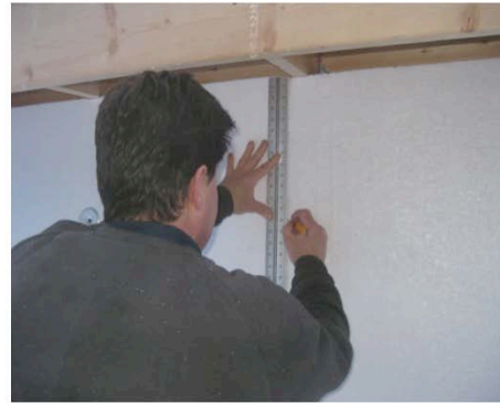
Trace stud measurement
