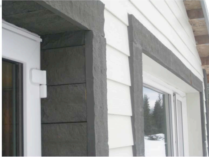
Inset style reduces heat loss and H 2 O that hits window
